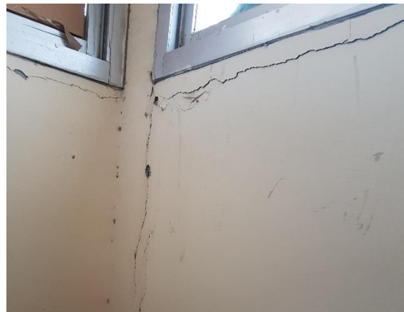
Fig. 6: Wall cracks
