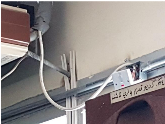
Fig. 5: Wiring defects
